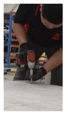
Assuming that the drilled hole is within the acceptable dimensions, the ease of installation is influenced by a number of factors. The top two main influencers are thread pitch+profile and steel strength + hardness.
